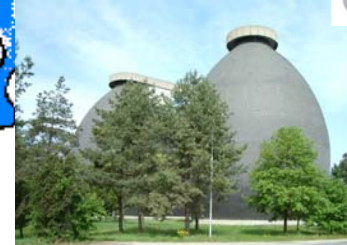
Linz, Austria , 1.500 hours operation (Waste water treatment plant in Asten, Linz AG)
