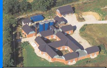
Owschlag, Germany , 2.200 h operation (Industrial research center, Seaborne GmbH)
