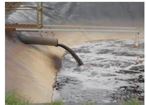
Landfill leachate entering retention ponds for treatment.
